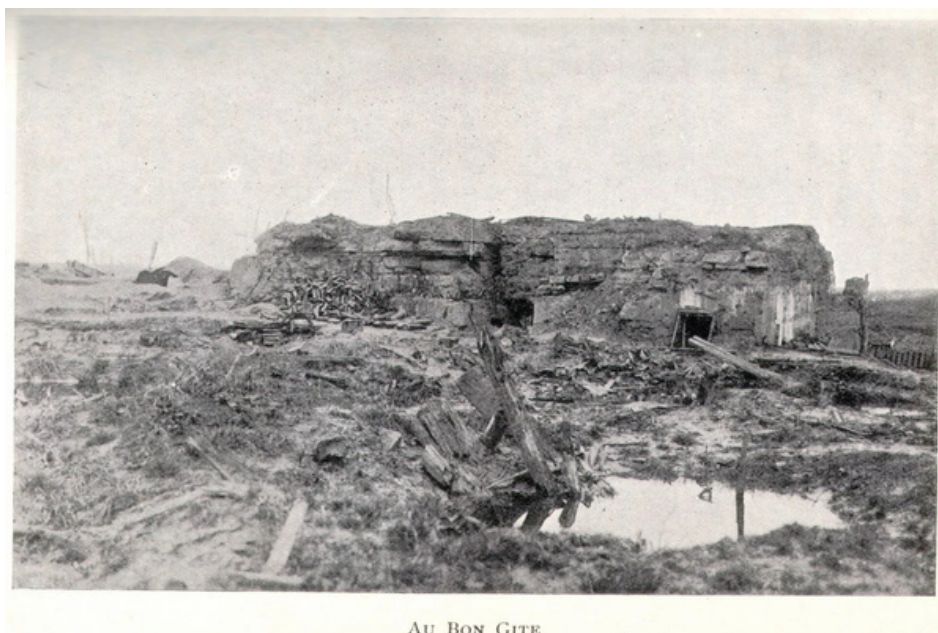
The German strongpoint Au Bon Gîte - a fortified concrete blockhouse
